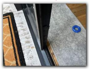
Damaged and missing weather stripping was noted at the master bedroom exterior door. The weather stripping should be replaced.
