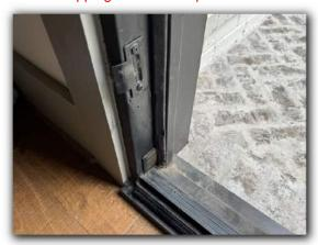
The dead bolt is difficult to operate at the master bedroom exterior door. All dead bolts should be adjusted to operate properly and easily.
