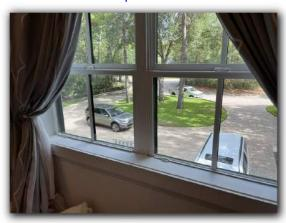
☑ Fall protection not provided for windows installed above 72" from grade. Fall protection is required at windows that are less than 24" from the finished floor and greater than 72" from the final grade. The fall protection is required to limit the opening of a window that meets these requirements so that a object 4" or larger cannot fit through the opening. This is safety hazard that should be addressed.
