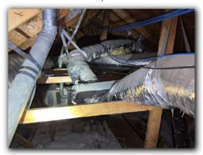
A disconnected vent pipe was found in the upper attic. It appears that this vent is not in use. However, it is recommended that it be verified that this vent is no longer in use or needed as I cannot locate the point of termination.
