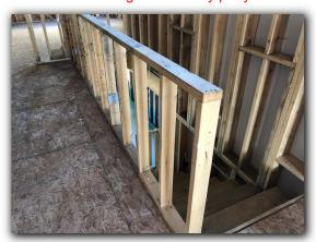
A damaged / broken sheer wall brace was found in the upstairs rear section of the home. Recommend repairs.
