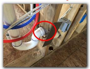
(R602.6), (R302.11) Fire / draft stopping missing in second floor air chase and garage wall areas of the structure.
