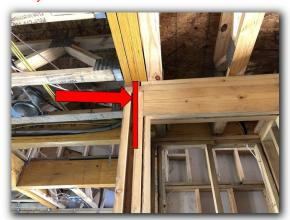
(R602.6) Exterior / Bearing wall stud drilled 40% - 60% not double and/or more then 2 successive studs located garage wall of the building.
