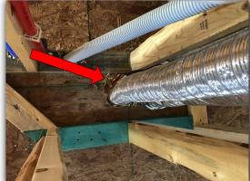
Recommend installing shims for wall sheer bracing were gaps are present.
