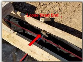
Beam tendons draped and secured by #3 rebar stakes or concrete bricks:  $\boxtimes$  Yes  $\square$  No Amble chairs all tied:  $\square$  Yes  $\boxtimes$  No
