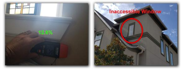
All exterior wall penetrations (electrical panels, electrical disconnects, light fixtures, etc.) and openings (expansion joints, windows, door thresholds, etc.) should be sealed with an approved material to prevent water penetrations into the wall cavities. Properly sealed exterior veneers help provide a barrier against the weather, insects, and enable environmental control of the interior spaces.
