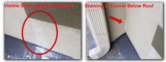
During the inspection of the wall and roof termination using a drone it was determined that kickout / diverter flashing had not been installed. It is suspected that this is one of the main causes of these extensive moisture problems.
