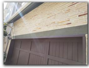
The transitions between differing materials have not been made properly. The transitions have been made with mortar which will eventually fail.
