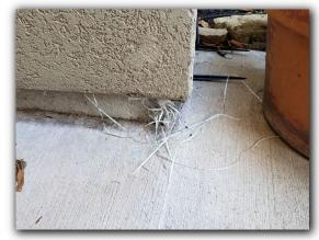
Failed sealant was found between the kickout / diverter flashing and the wall / roof termination.
