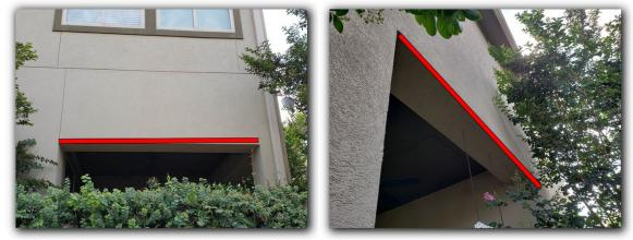
Improper clearance of the stucco was found at the back right porch column. Visible damage was found at this column.
