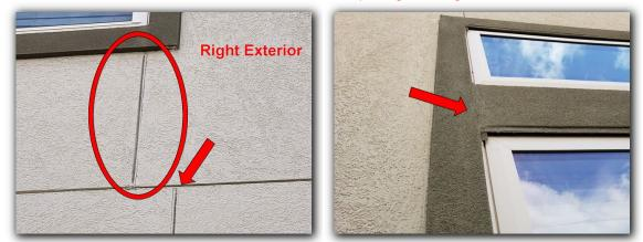
Missing mortar was found at the stone along the fence post on the right side of the home. This appears to have been not completed during construction.
