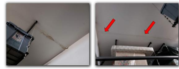
Slightly elevated moisture readings were found at the front right window on the interior. This area was inaccessible for invasive stucco probing. During repairs of the other areas this location should be evaluated and improved as needed.
