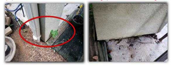
Improper clearance was found at the grade (soil), roof, and patio of flatwork.
