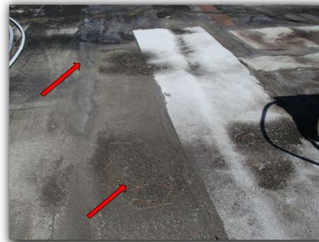
Worn asphalt was noted in areas of the flat roof coverings as evident by bare spots exposing underlying materials. Recommend further inspection/repairs by a qualified tradesman to prevent possible leaks.
