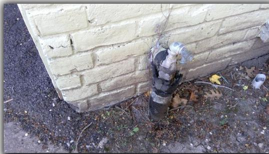
Active leaks should be repaired at the front right exterior of unit B15.
