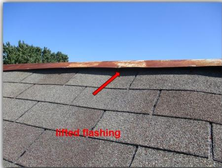
Raised shingles were found at the sections of the roof coverings. Recommend repairs by a qualified tradesman.
