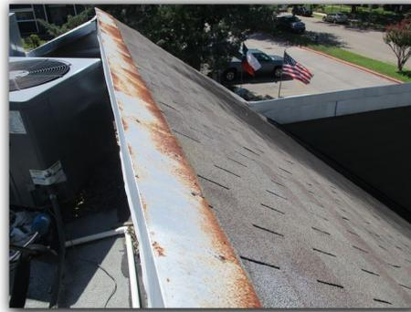
Sections of the roof flashings are raised which could lead to water penetrations. Recommend repairs.
