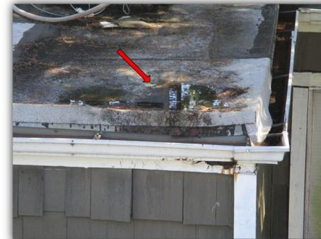
Wrinkling/blistering was noted in areas of the flat roof coverings. This can be caused by built up moisture and/or air under the roofing materials. Recommend further inspection/repairs by a qualified tradesman.
