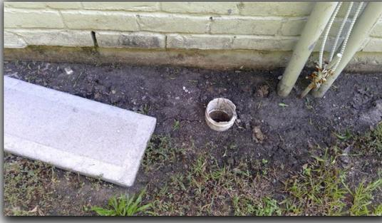
Standing water was found at the laundry room #2 exterior as evidence of improper plumbing drainage that may indicate underground breakage and or improper drainage. Repair by a licensed plumber is recommended.
