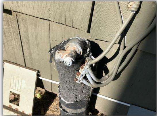
Many of the electrical meters are loose on the exterior wall of the buildings. The meter should be re-secured by a licensed electrician.
