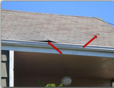
The lead / metal roof jacks have not been installed properly at some locations. The jacks do not completely cover the plumbing vents. These areas will be prone to water penetrations.
