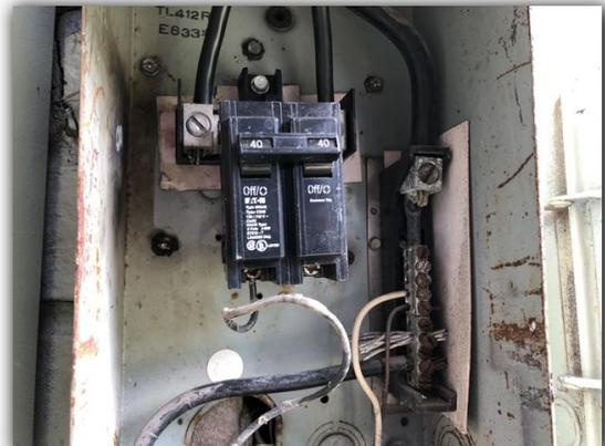
Aluminum wiring was observed at appliance breakers in several of the main service panels. The breakers are labeled for aluminum wiring but the connections at the receptacles for the appliances were not accessible to be inspected. Aluminum wiring must be fitted/connected with the special connectors and outlets to ensure safe operation of these circuits. Further investigation is recommended by a licensed electrician to verify that the aluminum connections are proper and perform repairs as needed.
