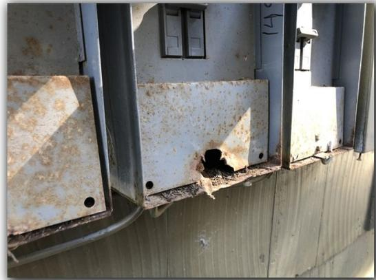
Many of the electrical panels are loose on the exterior wall of the building. The panels should be re-secured by a licensed electrician.
