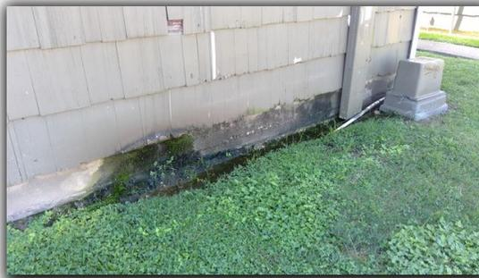
Missing gutter splashblocks should be installed at the base of the gutter downspouts to reduce soil erosion.
