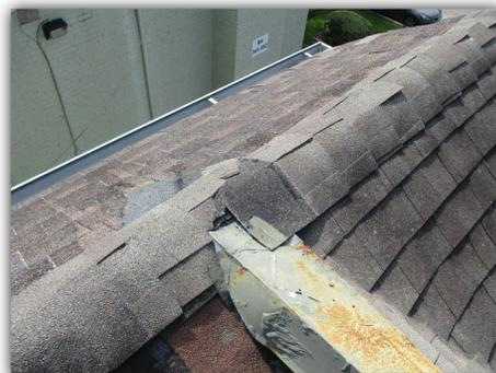
Exposed nail heads were found at roof jacks and / or sections of the flashings. All exposed nail heads should be sealed to prevent water penetrations.
