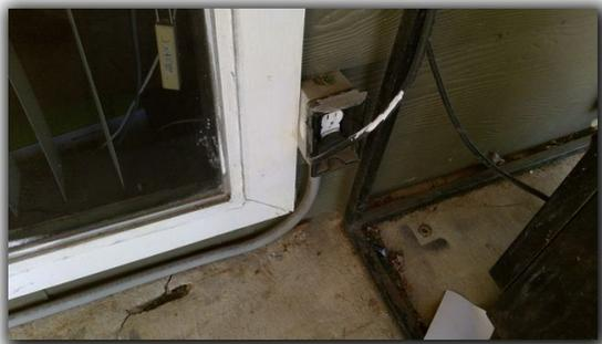
Missing globes, loose fixtures, and separated/loose conduit was found at many of the exterior lights/conductors.
