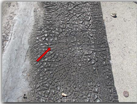
Soft spots were noted in a various locations on the rolled flat roofs. Soft spots on flat roofs could indicate rotted or improperly installed sheathing below the rolled roofing. A qualified tradesman should be contacted to inspect/repair the soft spots as needed.
