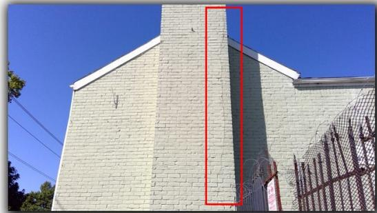
Diagonal cracking as evidence of potential differential movement
