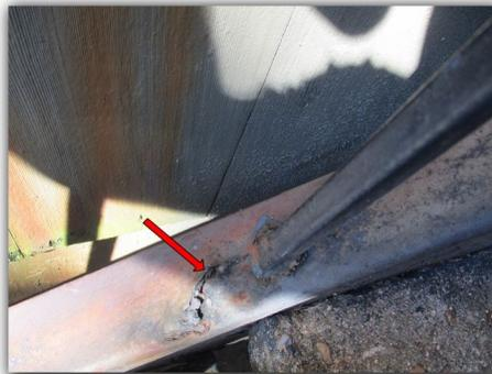
Rust, corrosion, damage and missing items were found at many of the handrails/balusters of exterior stairs. All rust should be removed to help prevent any future problems that may occur.
