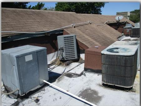
The refrigerant line dryer(s) at the exterior portion of the air conditioning system(s) are rusted at some units. These components should be inspected annually, cleaned and repainted to prevent leaks and other problems from developing. In addition, rust and corrosion was also noted on several of the units.
