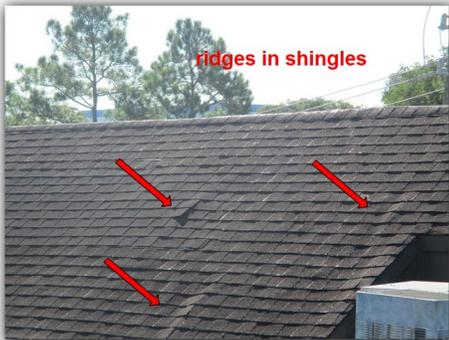
Damaged and / or missing shingles were found during the inspection of the roof coverings. Recommend repairs by a qualified tradesman.
