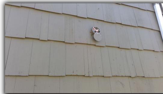
Receptacles at the exterior of unit # B13 are not functioning. Recommend further investigation and repairs by a licensed electrician.
