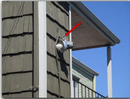
Improper electrical connections were noted on the roof of Building 6. Improper electrical connections should be improved. All electrical connections should be made inside junction boxes fitted with cover plates.
