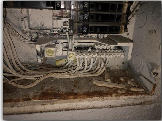
Many of the breakers within the panel boards have not been completely labeled. All circuits should be properly labeled.
