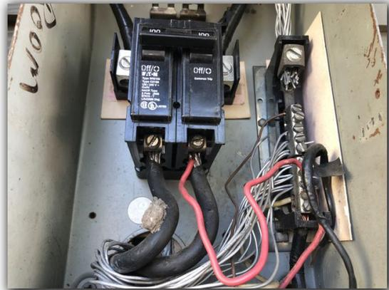
Oversized breakers were found within the electrical panel. Each breaker is rated for a specific size conductor. Ideally, these breakers should be re-sized by a licensed electrician.
