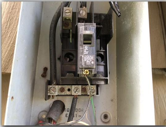
Most of the service box shows evidence of rusting, suggesting the presence of moisture. Many of the main electrical boxes are possible in need of replacement. Recommend further evaluation / replacement by a licensed electrician.
