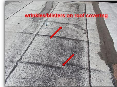
Alligatoring was noted on areas of the flat roof coverings. This can be caused by the sun's UV rays that dry out any type of exposed asphaltic roofs. These areas should be monitored and repaired as needed to prevent future problems with the roof coverings.
