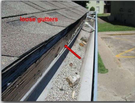
Leaky & damaged gutters were found around the perimeter of the roof coverings. The leaks should be repaired along with any damage caused by the leaks. It appears that multiple areas of damage have been caused by the leaking gutters. Repairs of the gutter / downspout systems as well as associated damages by qualified tradesmen is recommended.
