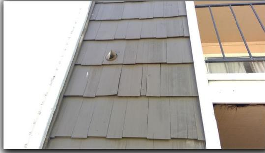
All exterior wall penetrations (electrical panels, electrical disconnects, light fixtures, etc. ) and openings (expansion joints, windows, door thresholds, etc. ) should be sealed with an approved material to prevent water penetrations into the wall cavities. Properly sealed exterior veneers help provide a barrier against the weather, insects, and enable environmental control of the interior spaces.
