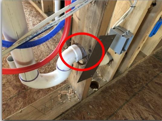
(R602.6), (R302.11) Fire / draft stopping missing in second floor air chase and garage wall areas of the structure.
