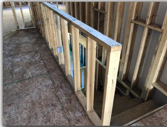
A damaged / broken shear wall brace was found in the upstairs rear section of the home. Recommend repairs.
