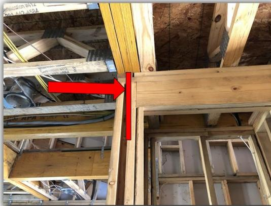
(R602.6) Exterior / Bearing wall stud drilled 40% - 60% not double and/or more then 2 successive studs located garage wall of the building.
