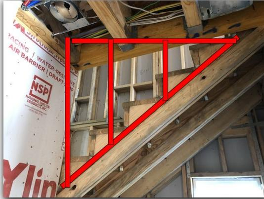
Missing stud under the triple ceiling joist. Generally, each joist beam has a stud for support directly below.
