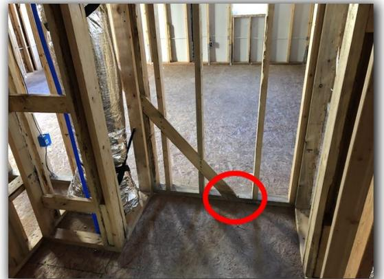
(R703.3.2) Exterior wall covering not fastened properly to manufactures specifications.
