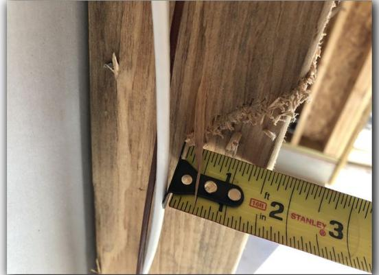
(R403.1.6) Anchor bolts or straps missing and/or improperly spaced on exterior wall. (At least 6 feet spacing and 12 inches from end of plate.)
